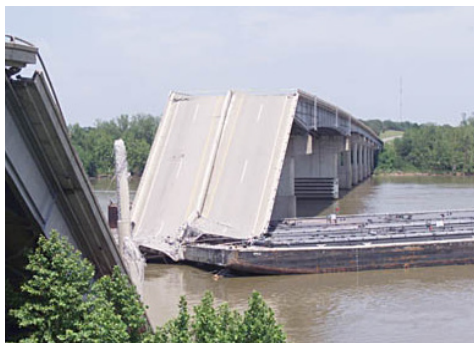
Figure 1. I-40 bridge collapse due to barge collision at Webbers Falls, OK (2002) (Photo credit: Oklahoma Department of Transportation)
